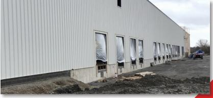
Having used FORTA-FERRO in several other buildings, owners chose to replace specified steel reinforcement in this newly constructed building. This allowed contractors to speed up pouring of the concrete and created a safer job site. This macro synthetic fiber also establishes a **better wearing surface** over the life of the concrete.
