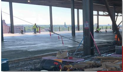
This newly constructed multi-story building used FORTA-FERRO macro synthetic fibers in lieu of welded wire fabric. This eliminated the space needed to store and the time need to place WWF. The Preferred Contractor, Barton Malow, uses FORTA's most popular fiber reinforcement in all project possible.
